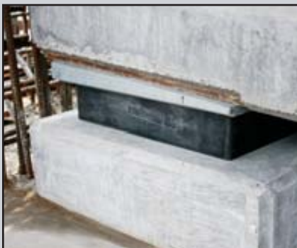
Bearing – Series EL with beveled top plate
