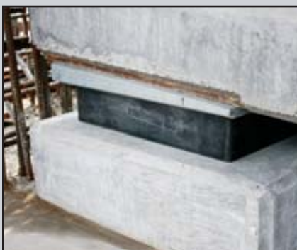
Bearing – Series EL with beveled top plate
