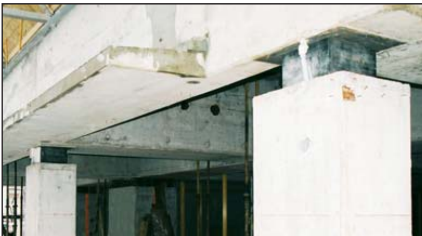
Twenty Gothic Condominiums, Toronto, ON
